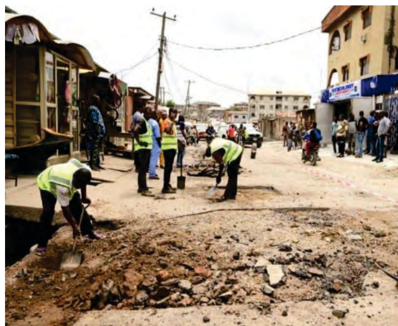
Rehabilitation work in progress
